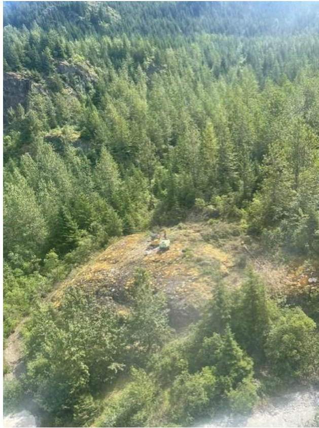
Fig. H: Aerial view of construction work at meteorological tower site
