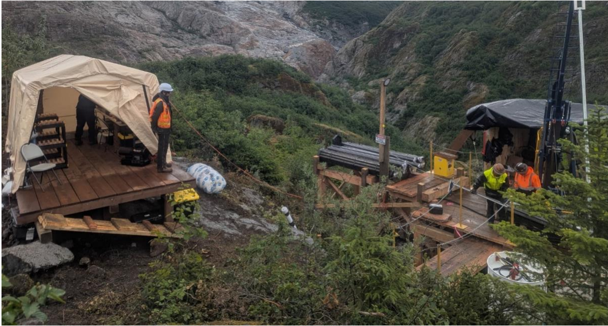
Fig. B: Drilling operations
