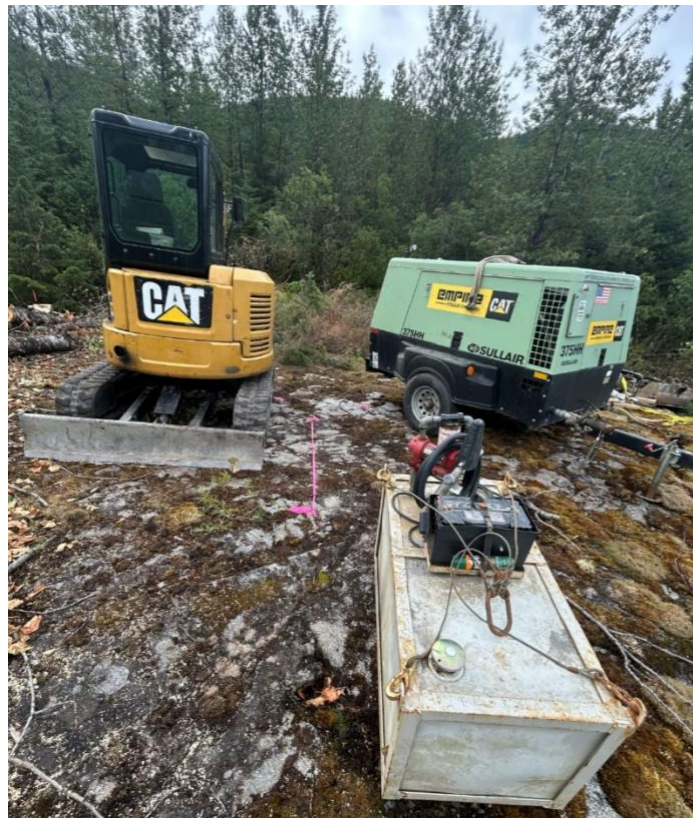
Fig. I: Construction equipment transported by helicopter to meteorological tower site
