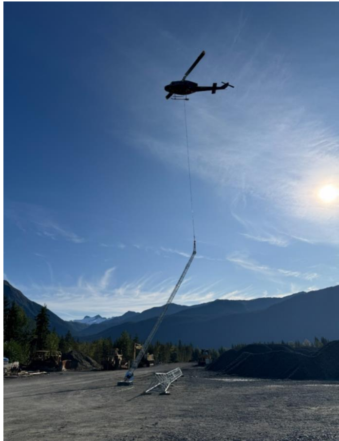
Helicopter transport of meteorological tower superstructure to project site
